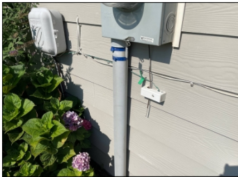
Electrical service meter grounded
