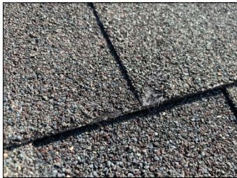
Normal wear to the shingles was observed
