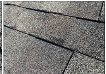
Normal wear to the shingles was observed. If concerns are present have a roofing contractor evaluate the roof and repair/replace components as needed.
