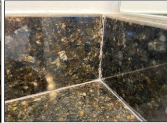
Primary bathroom counter sealant has gaps
