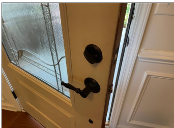
Front door not latching properly and the deadbolt not engaging the frame easily
