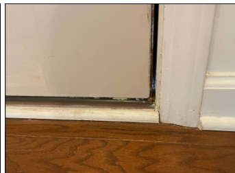
Door not sealing at the lower corner
