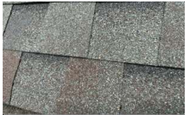
Shingle Condition - Granular attachment typical and consistent with age of roof.
