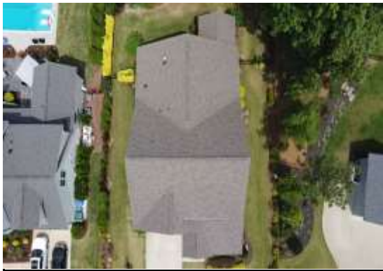
Overall Roof Photo
