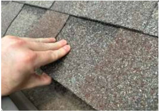
Shingle Condition - Granular attachment typical and consistent with age of roof.
