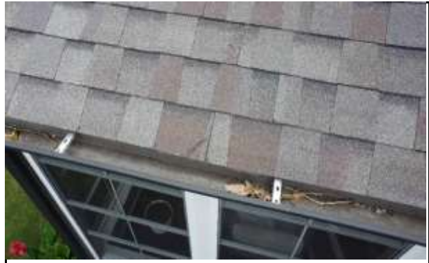
Gutters - Gutters are properly attached and function as intended/good shape
