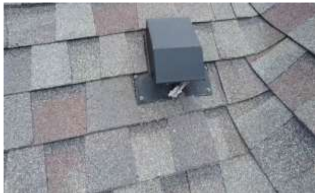
Mechanical Flashings - Mechanical flashings are in good shape. These flashings are recommended to be replaced every 8-10 years.
