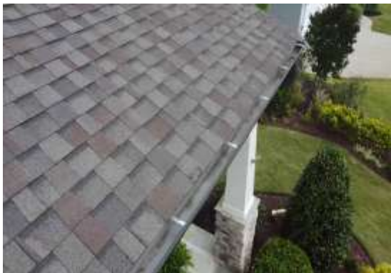
Gutters - Gutters are properly attached and function as intended/good shape
