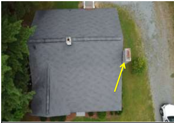
Aerial View (Chimney Location) Photo 1 NR
